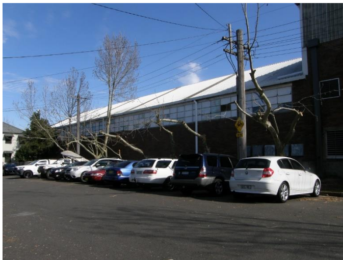
Figure 19 – View of the Fred Street elevation. (NBRSArchitecture, August 2016)
