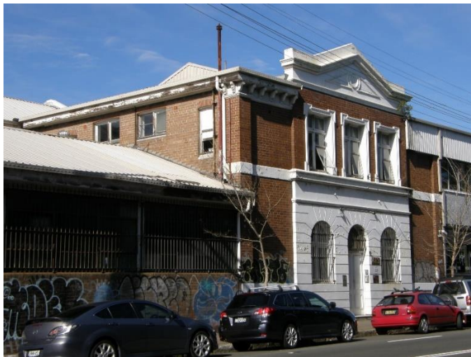
Figure 31 – General view showing the return wall of the office entrance. (NBRSArchitecture, August 2016).
