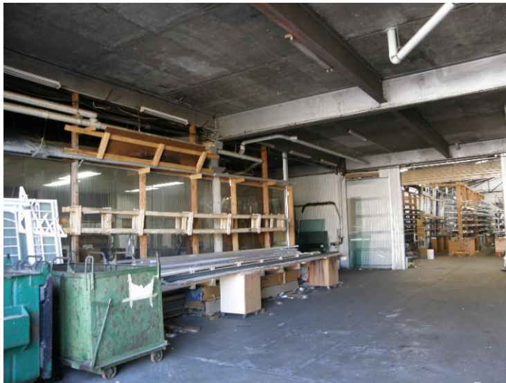
Figure 39 – General view of ground floor warehouse interior. (NBRSArchitecture, August 2016)
