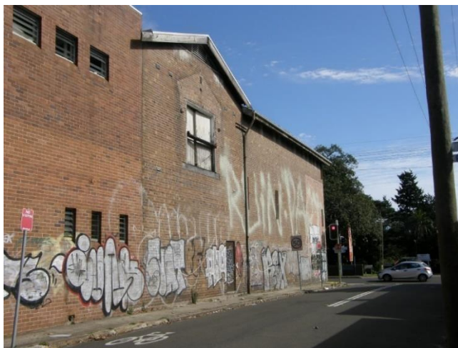
Figure 22 -Part view of the Cecily Street elevation showing the extent of the original Pilchers Baking Company building, and evidence of an earlier roof and hoist over the first floor doors. (NBRSArchitecture, August 2016)
