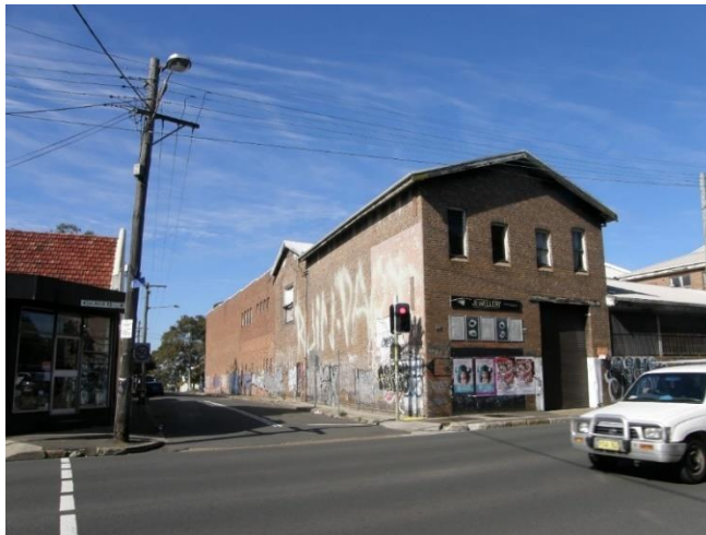
Figure 21 - View of the Cecily Street elevation of the former Pilchers Bakery Company Factory. (NBRSArchitecture, August 2016)
