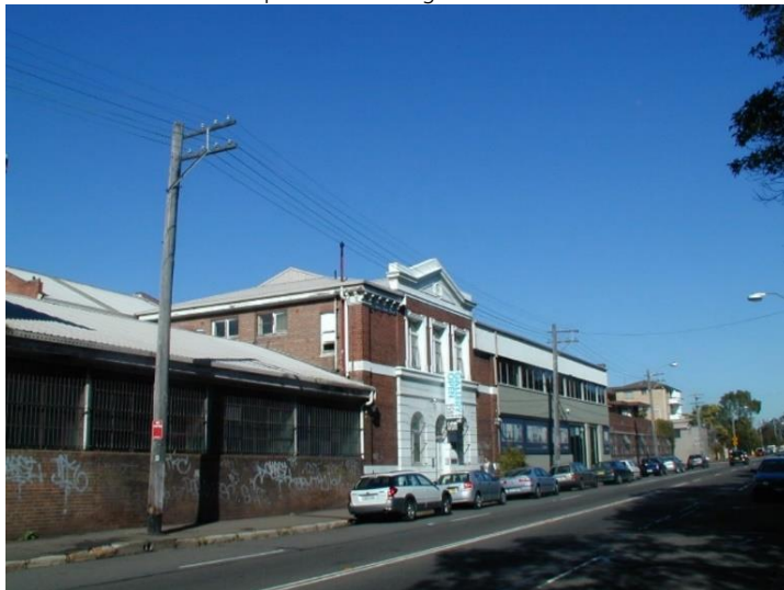
Figure 29 – View of the Balmain Road elevation of the former factory development. (NBRSArchitecture, August 2016)
