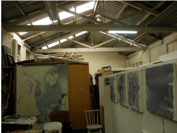
Figure 26 - Typical timber roof trusses and metal roof over southern section of the former Pilchers Baking Company building. (NBRSArchitecture, August 2016)
