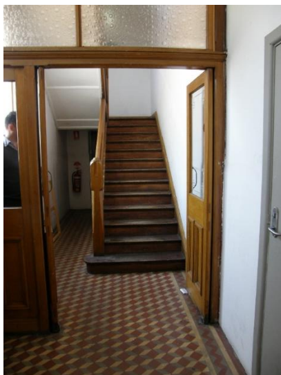
Figure 32 - Part view of the original stair and tiled foyer area. (NBRSArchitecture, August 2016)
