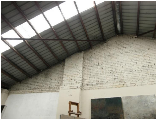
Figure 34 - View of the first floor interior showing the rendered wall finish and the location of the original ceiling. (NBRSArchitecture, August 2016)
