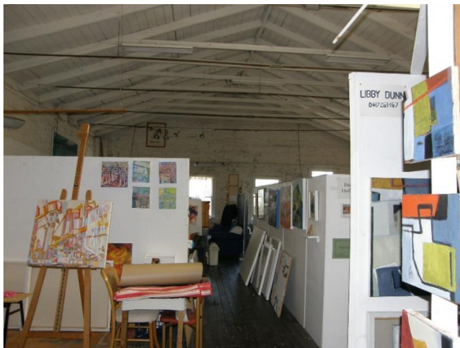
Figure 24 - Interior of the northern section of the former Pilchers Baking Company building showing the raked boarded ceiling, metal rod bracing and timber floors. (NBRsArchitecture, August, 2016)
