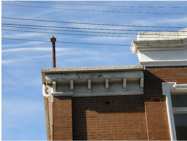
Figure 30 - Eaves bracket detail. (NBRSArchitecture, August 2016).
