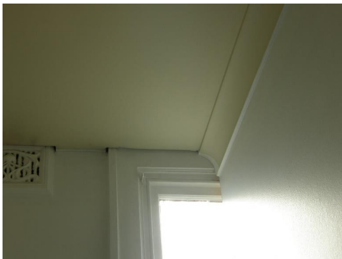
Figure 35 - Detail of a first floor space showing a new stud wall located adjacent to an existing window. Note the new plasterboard ceiling cut around the window architrave and wall vent. (NBRSArchitecture, August 2016)
