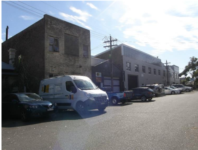
Figure 13 - View looking north west along Fred Street, Lilyfield, showing the surviving factory and warehouse buildings. (NBRSArchitecture, August 2016)
