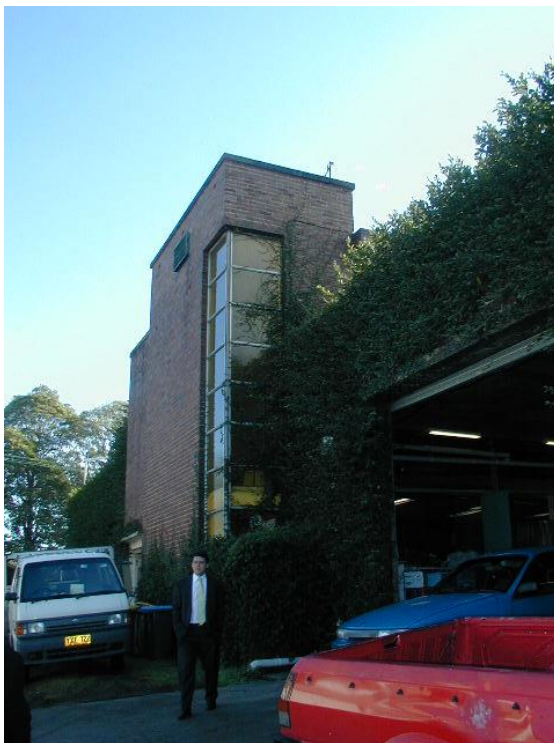
Figure 37 - The Alberto Street entry and stair tower to the rooftop residences. The elevation is now covered with vegetation and the brickwork is not visible. (NBRSArchitecture, 2006)
