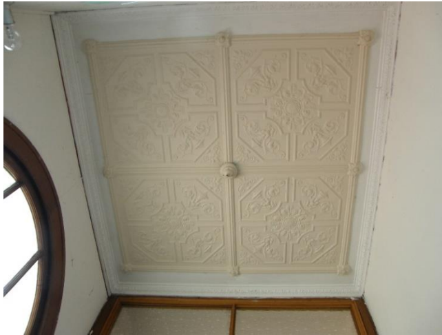
Figure 33 - Detail of the surviving section of pressed metal ceiling in the entrance foyer. (NBRSArchitecture, August 2016)
